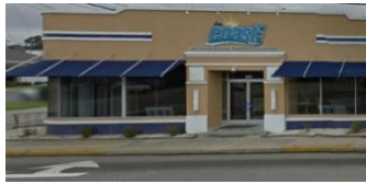
Conway Terminal 1418 Third Avenue Conway, SC
