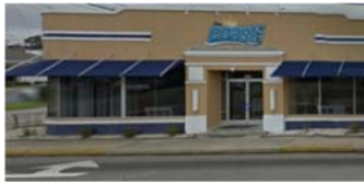
Conway Terminal 1418 Third Avenue Conway, SC
